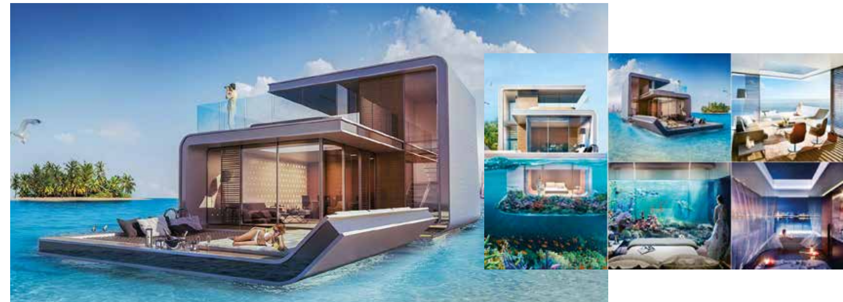
The Floating Seahorse villas (42 villas), Dubai, U.A.E.
